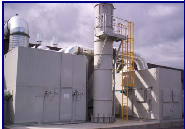
36,000 SCFM Concentrator with Catalytic Oxidizer system installed at an Oregon facility.
